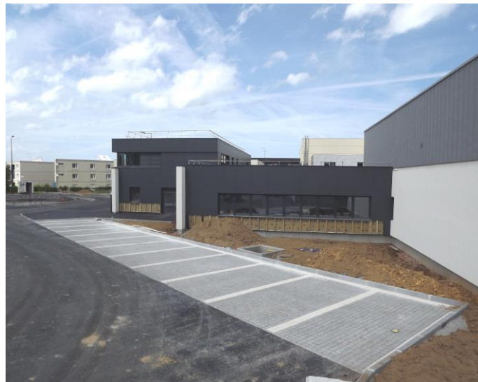
Fig 2. Parking spaces made with pervious concrete pavers – ESITC Caen, Epron, France
